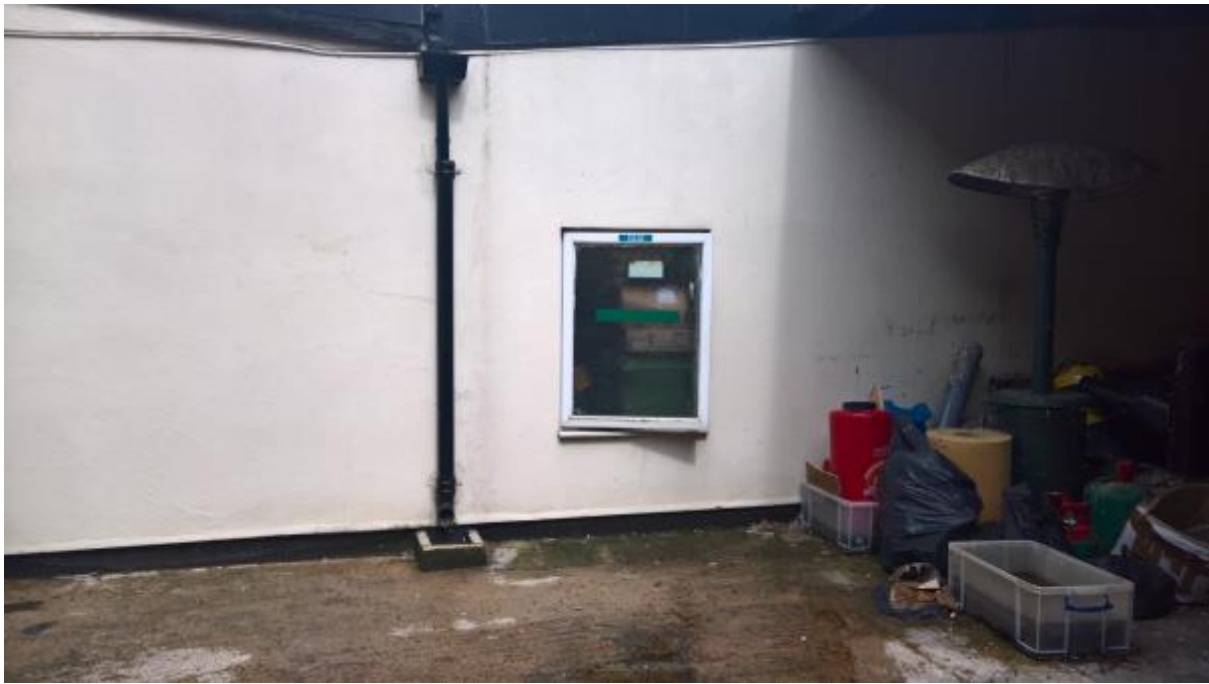
Rescue opening in the court yard for No 1A Gloucester Place
