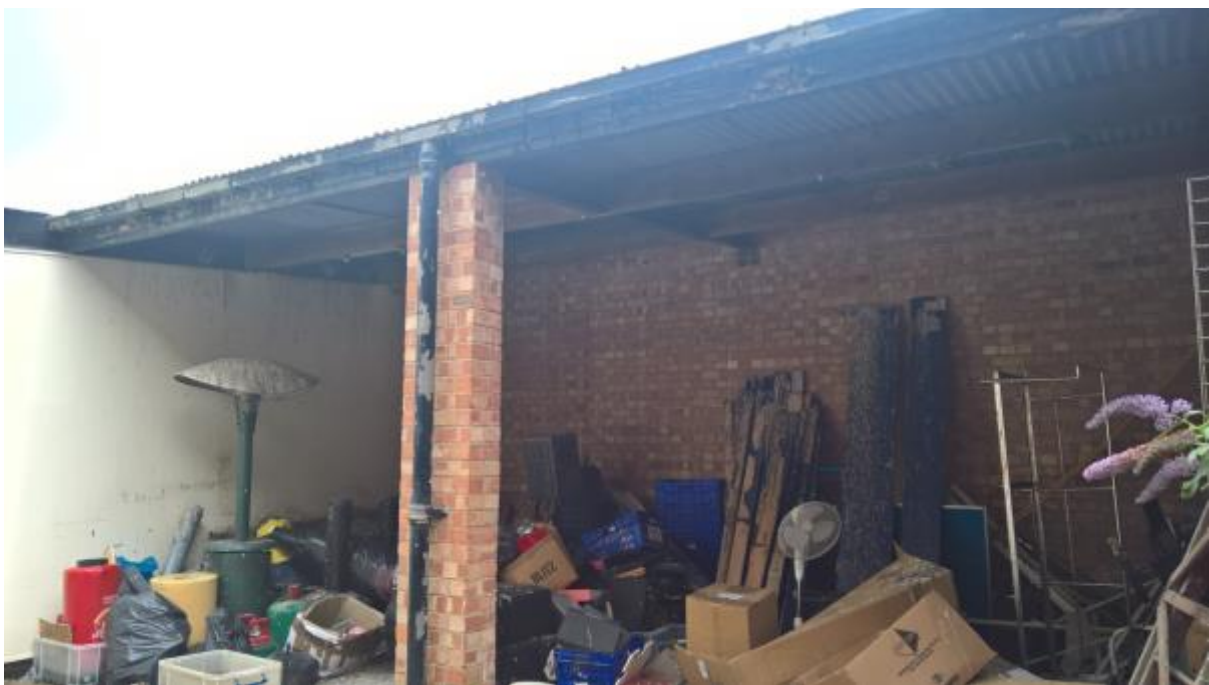
Court yard shed
