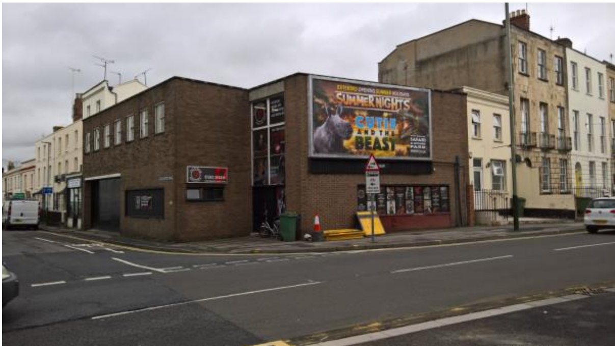
Corner view of Albion Street and Gloucester Place
